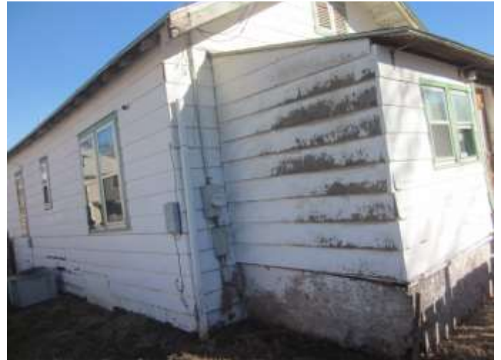
View along west side
